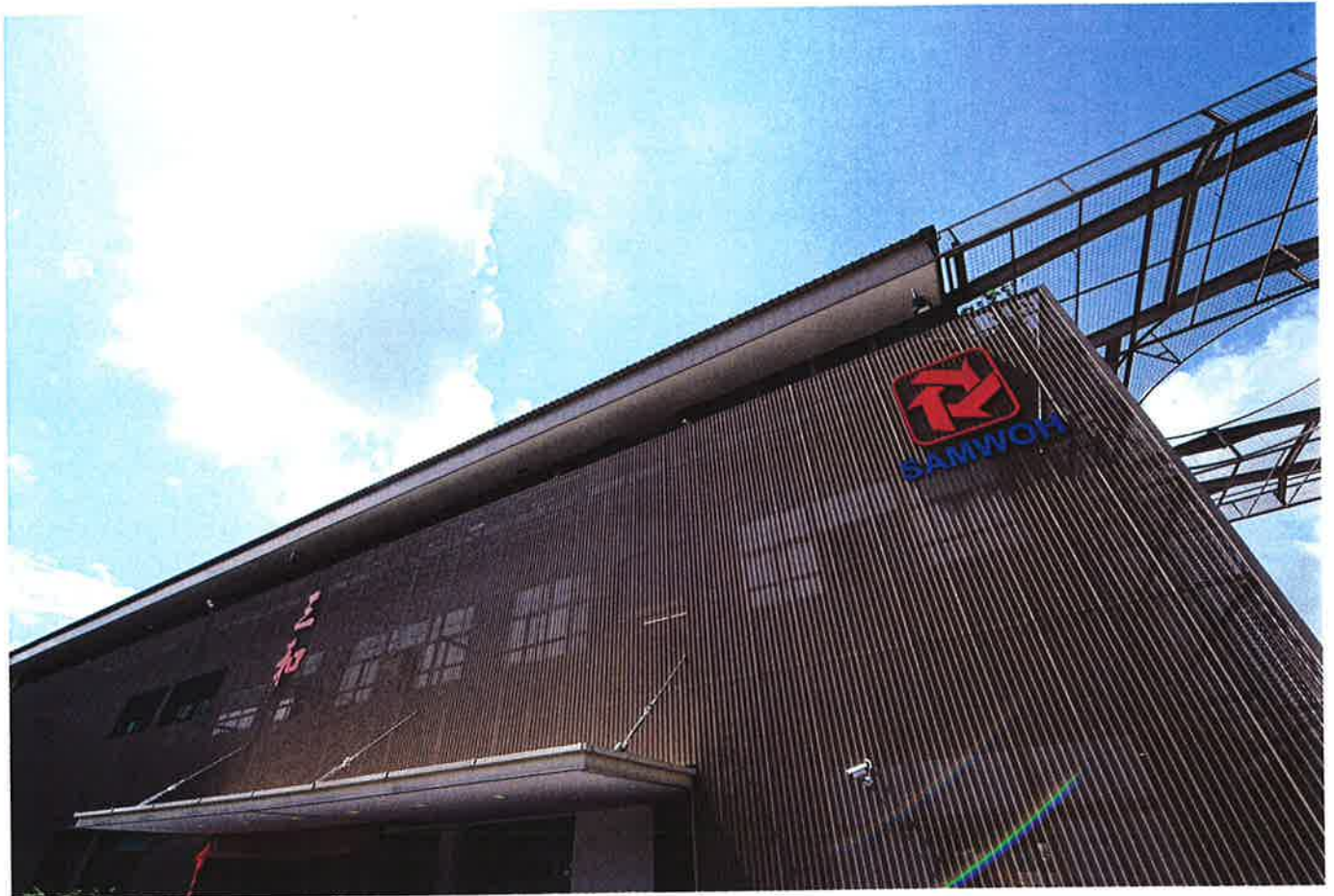
SAMWOH CORPORATION'S ECO-BUILDING IS THE FIRST PROPERTY IN SOUTHEAST ASIA TO BOAST AN ENTIRE LEVEL BUILT WITH CONCRETE CONTAINING 100 PER CENT RECYCLED AGGREGATE (LOOSE GRANITE). THE BUILDING LOCATED IN THE INDUSTRIAL ESTATE OF KRANJI CRESCENT IS COVERED IN A STEEL MESH TO PROTECT IT FROM THE SUN AND DUST.
