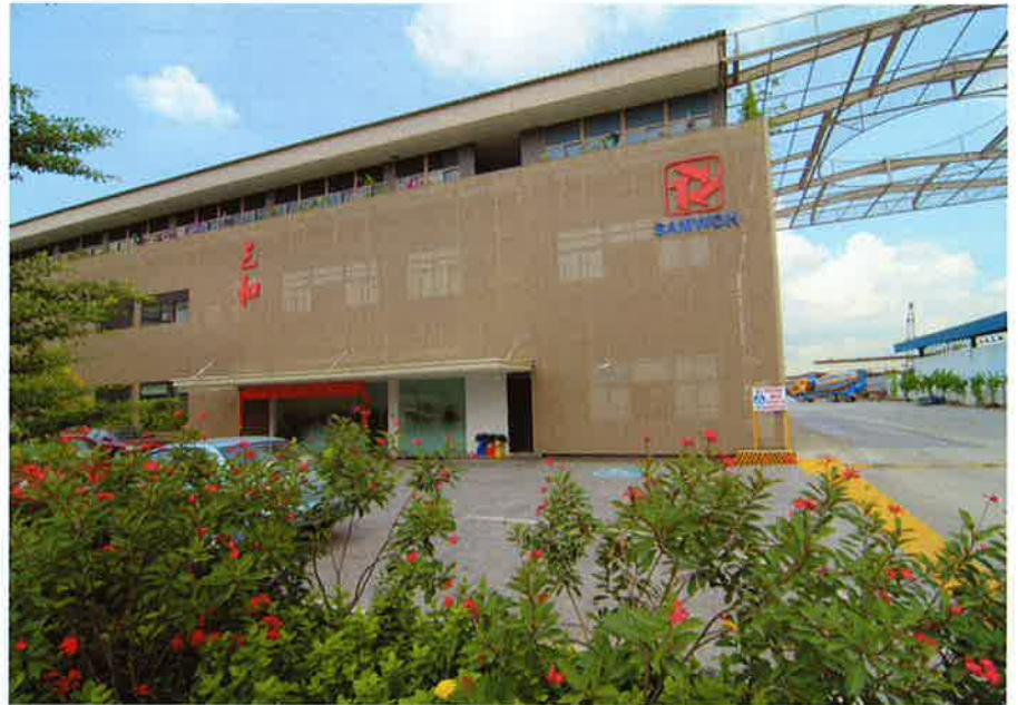
The Samwoh Eco-Green Building.
