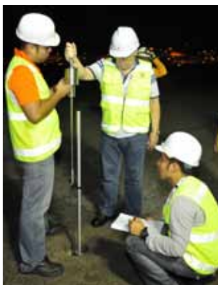
In-situ California Bearing Ratio (CBR) Test
