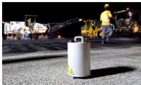
Testing of Pavement Surface Macrotexture
